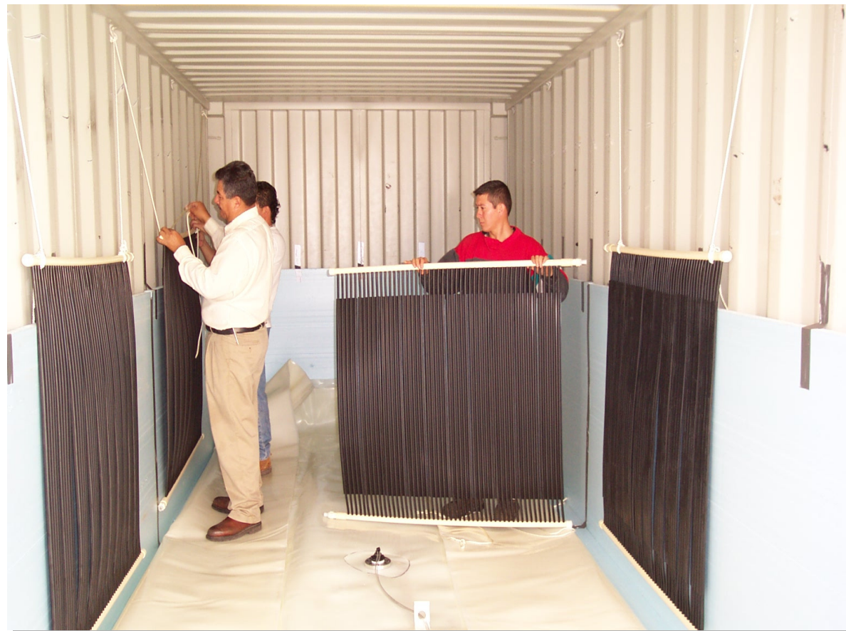
Side-wall heater units
